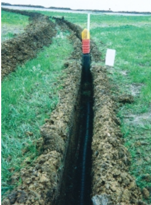
ADS pipe helps complete an efficient terrace drainage system.
