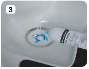
Pour about <u>30 oz. of water</u> over the Drain Insert. Then slowly pour the <u>entire contents</u> <u>of the Odor Barrier</u> onto the Drain Insert. Wipe clean. The American Standard Urinal is now ready for use.
