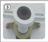
Remove old rubber gasket and clean flange and drain thoroughly. Install NEW FLANGE COUPLER, rubber gasket with longer part towards the wall and tighten bolts.
