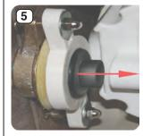
Hang the Urinal. Check for pitch and alignment to waste line pipe. Adjust Wall Bracket up or down as needed for proper drain line pitch and alignment.
