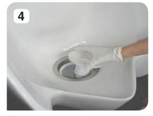
Take a new Drain Insert and place it in the waste trap.
