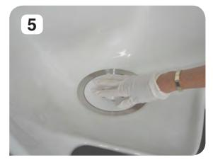
Press down on the Drain Insert until you feel and hear a slight popping sound. The insert must be tight.
