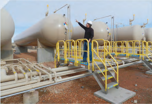
30" vertical clearance, 9' span over pipes.
