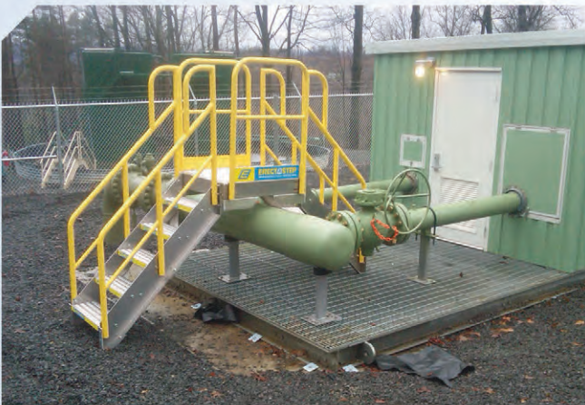
Pump station access was an afterthought.
