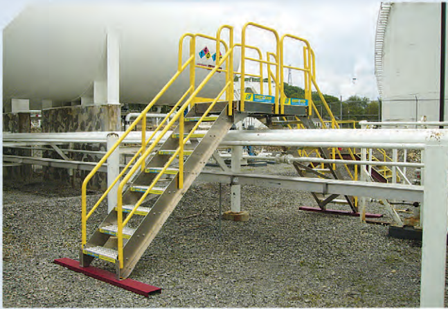
Eight stair pipe crossover.
