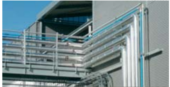
Outdoor installation Transair Ø 168
